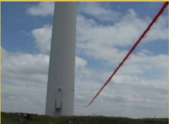
Location: Germany, wind farm
